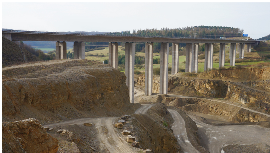
Figure 11. Highway bridge partly founded in a mining site.
